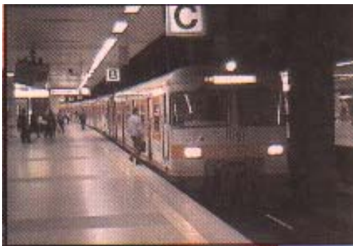
Laser control system to watch the platforms in underground stations (General Electric)
