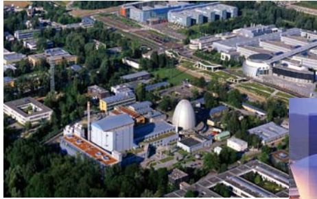
The new Research Reactor FRM-II at Garching, GER
